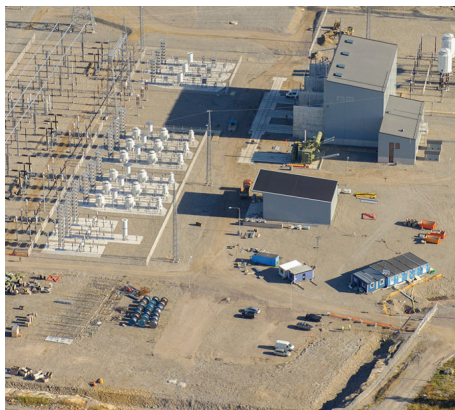
Anttila converter station
