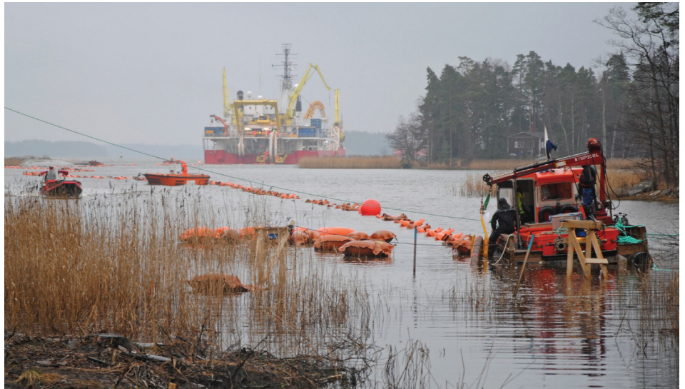
Submarine cable installation in November 2012 in Finland
