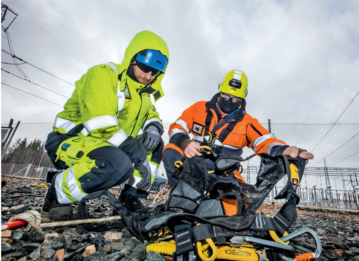
The first trial climb took place in May at the Keminmaa substation. Pictured: electrician John Salonen (left) and Esa Kärnä of Kärnä Oy, a consultant on the project focusing on working at height.
